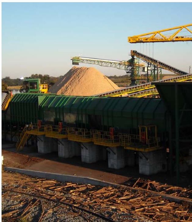
Rockwood stacker-reclaimer (center) at Packaging Corporation of America's Valdosta, Georgia, facility.
