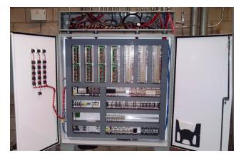
The OptoEMU Sensor and other SNAP PAC System hardware is wired to SUPERVALU's refrigeration system components and gathers consumption data. This data is then made available to both the company and curtailment service provider Net Peak.
