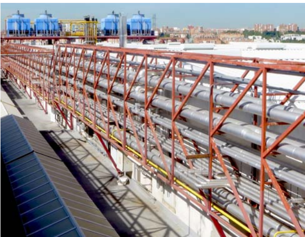
Liquefied ammonia, ethylene glycol, and other fluids are pumped throughout the market using a pipeline manifold equivalent to 43 mi. (70 km).
