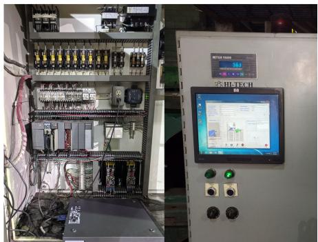
One of the previous feeder system electrical panels and HMIs, circa 2000
