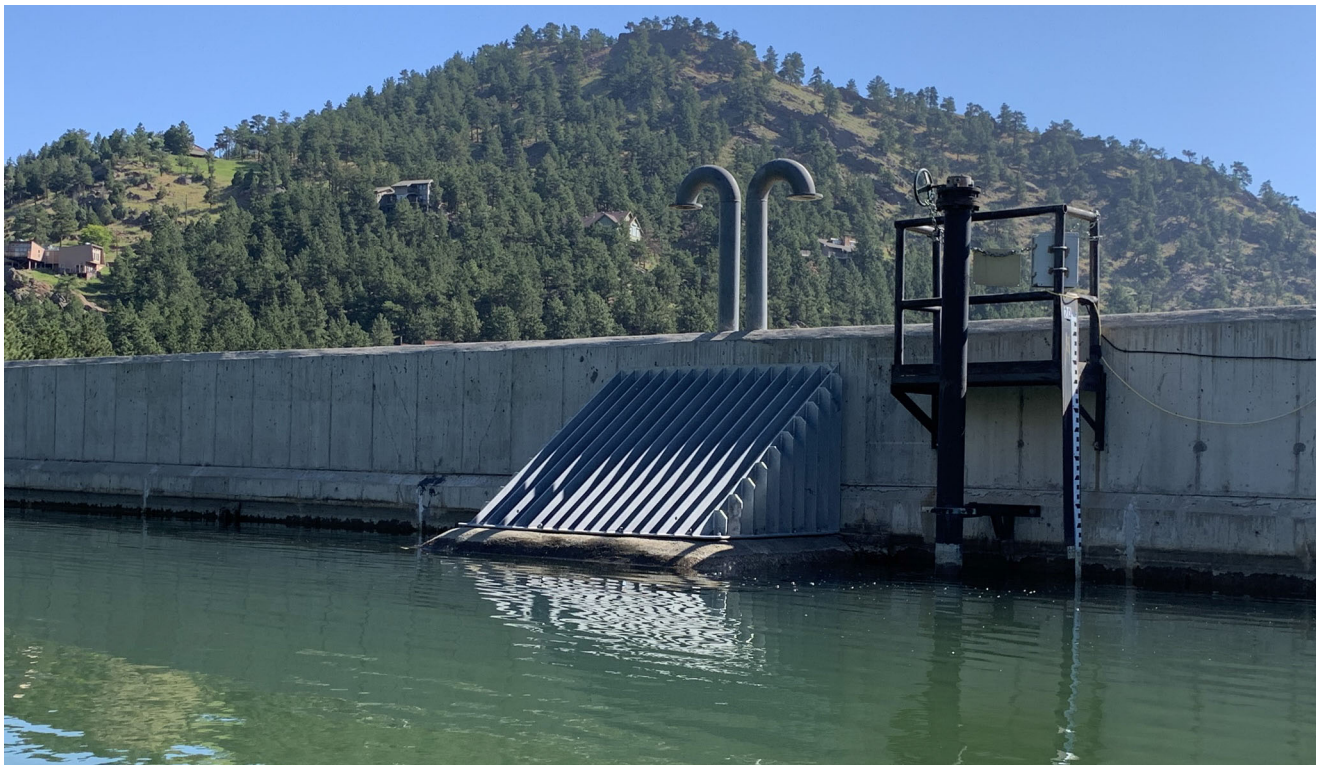
The Pinebrook Water District reservoir lies in the hills northwest of Boulder, Colorado.
