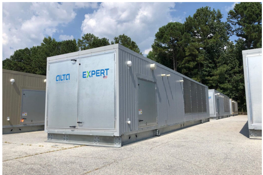
Each EXPERT follows a standard, reliable design that can be mounted on the roof above the area it serves.
